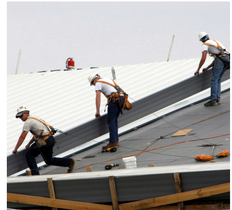
Cool roof installation
