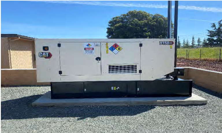
E. Recreation Center Emergency Generator Project
