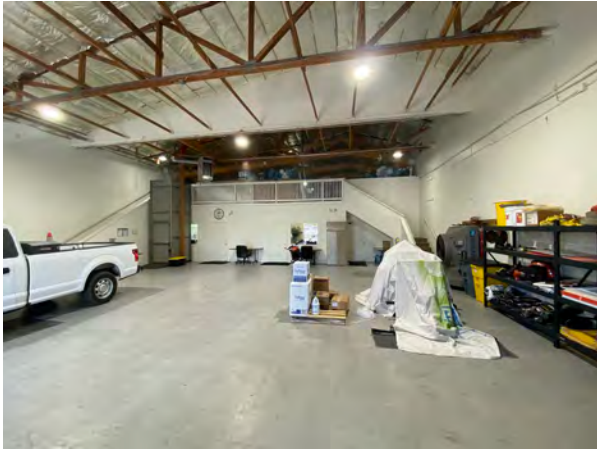
M. Public Works Operations Building Remodeling Project
