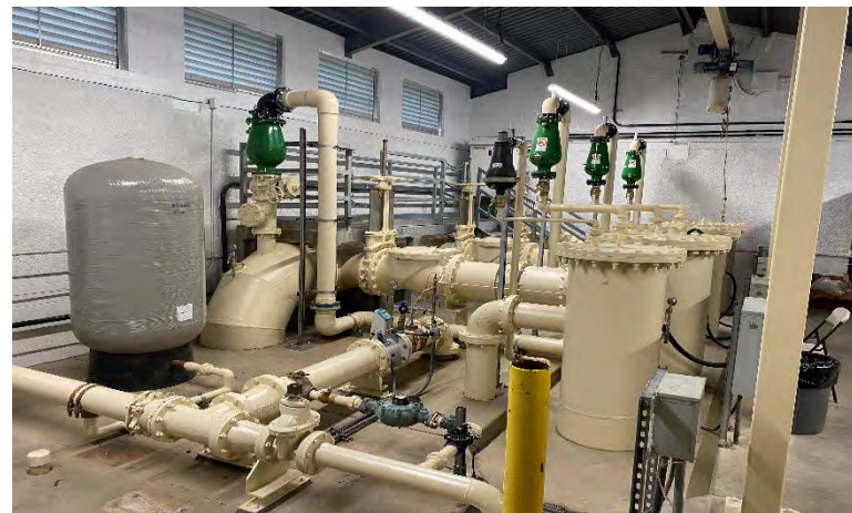
F. Cypress Grove Subdivision Pump Station Building Project
