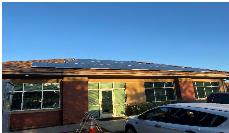
H. City Hall Rooftop Solar Power Project
