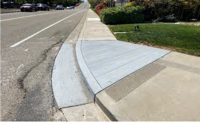
K. FY 2023/24 Curb, Gutter, and Sidewalk Repair and Reconstruction Project
