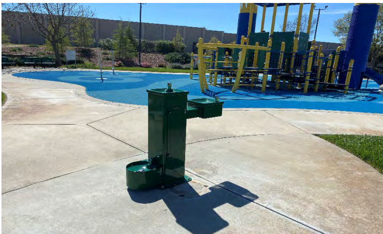
P. City Parks Drinking Fountain Replacement Project
