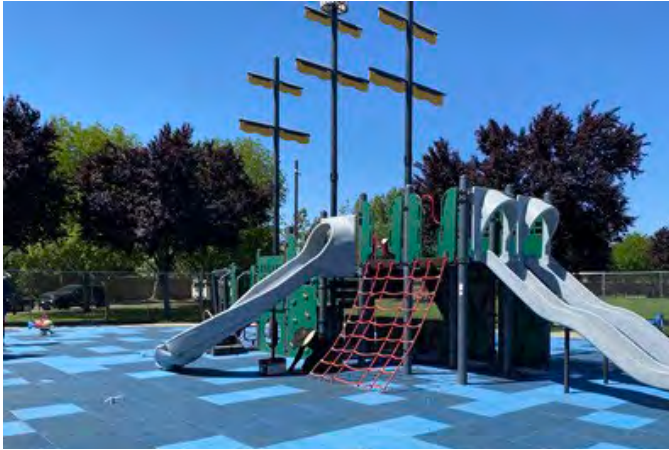
O. Daffodil Park Playground Resurfacing Project
