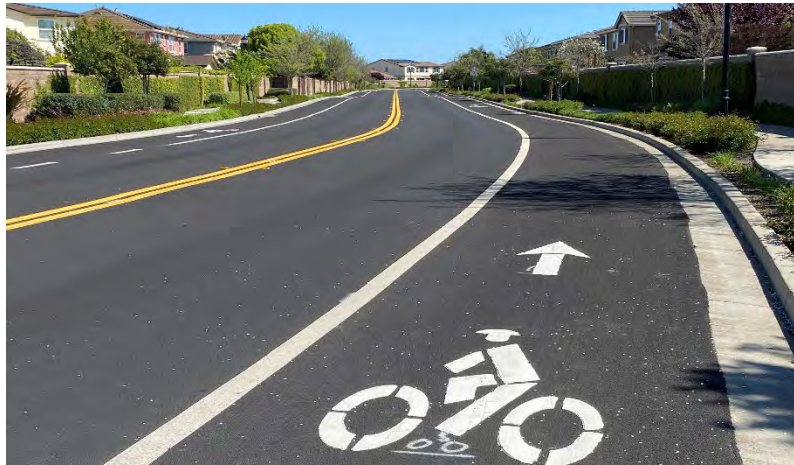
G. FY 2022/23 Street Repair and Resurfacing Project
