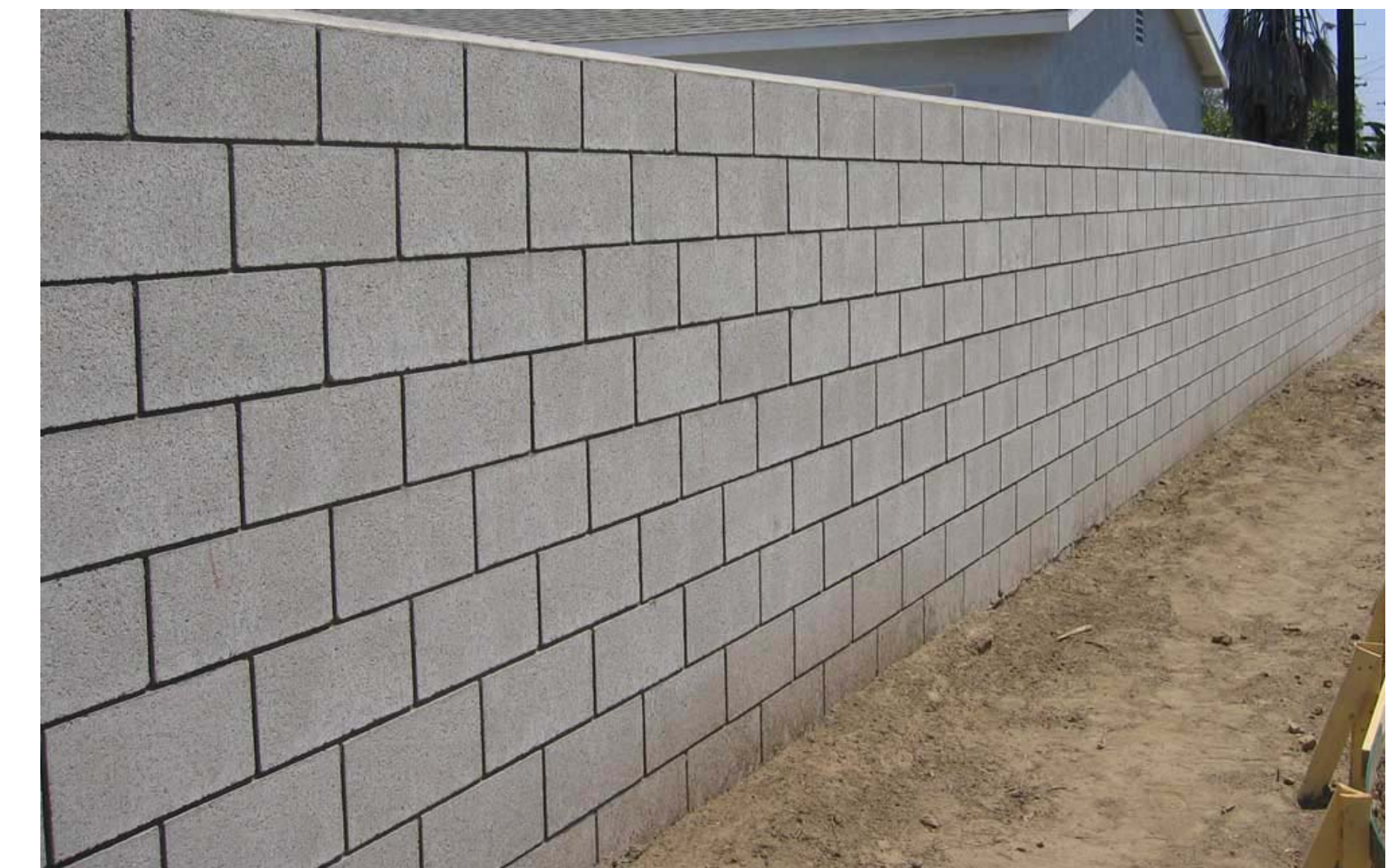
Masonry Wall at North Property Line
