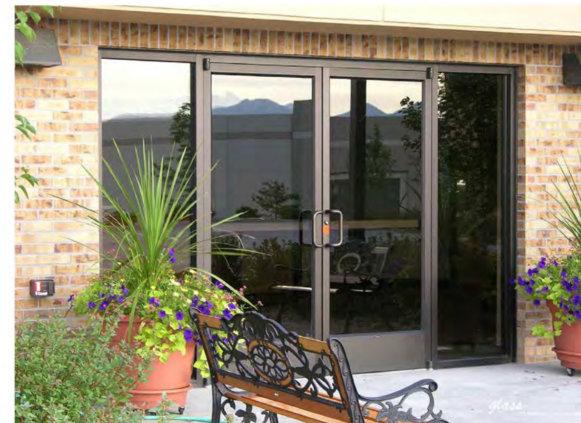
STOREFRONT SYSTEM - (EXAMPLE IMAGE ONLY) DARK ANODIZED ALUMINUM AMERICAN GLAZING & ALUMINUM INC. OR APPROVED EQUAL
