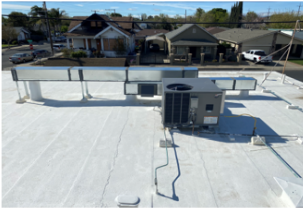
D. Senior Center Roof & HVAC Replacement Project
