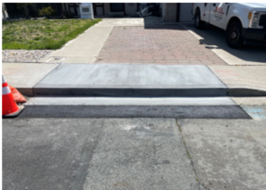
E. Curb, Gutter, & Sidewalk Repair Project
