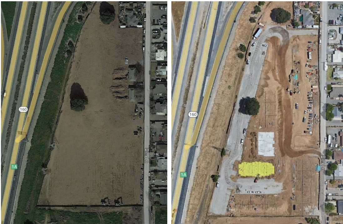
Before (February 2022) and after (March 2023) aerial images of the Elm Lane/Anton multi-family project.
