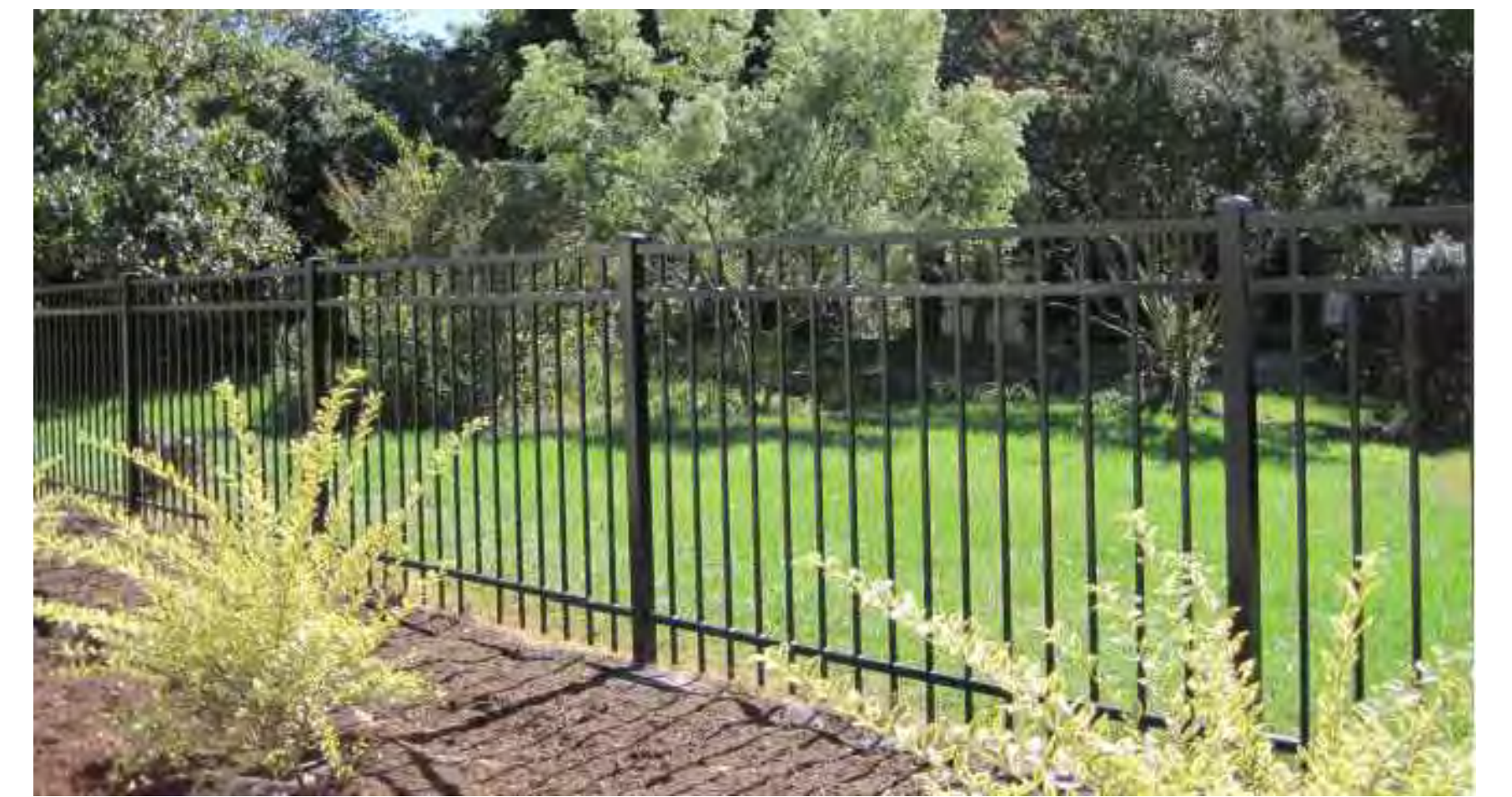
C 6' HIGH TUBE STEEL FENCE
