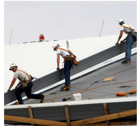
Cool roof installation
