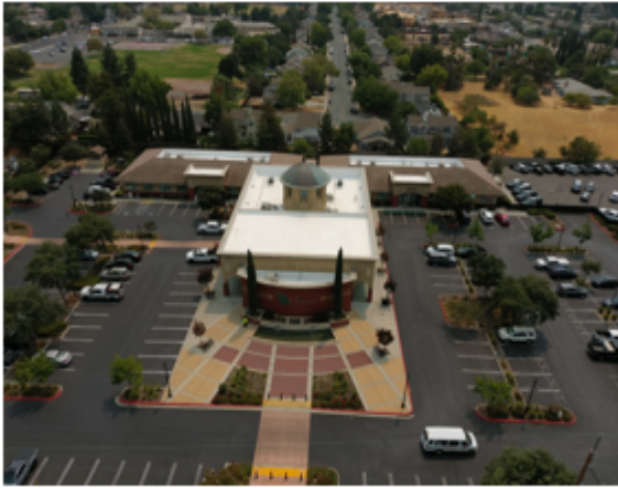
F. Civic Center Roof Replacement Project
