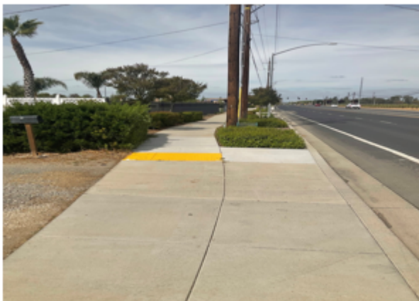
E. Curb, Gutter, & Sidewalk Repair Project
