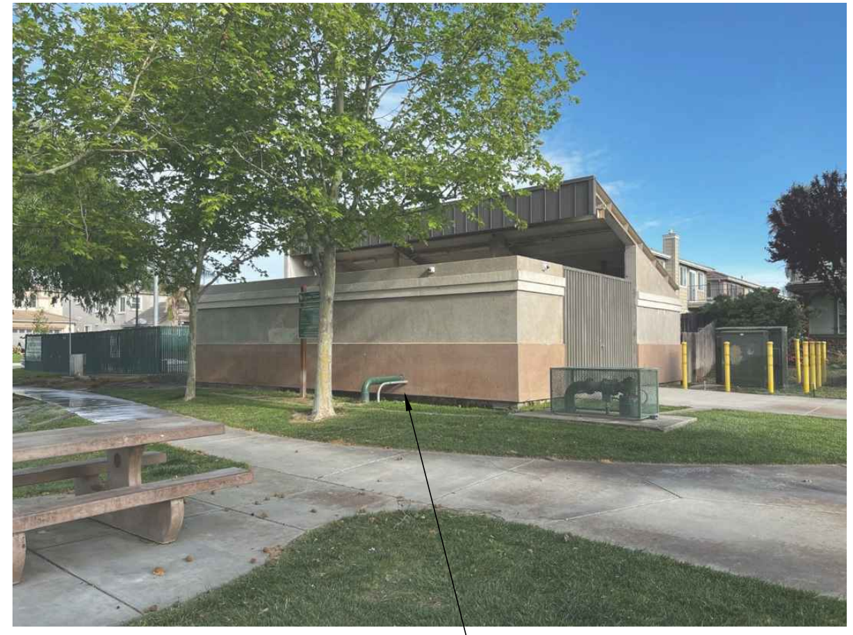
20. REBUILD WELL PIPE INSIDE OF THE BUILDING. REROUTE CONDUIT ALONG SOUTH WALL INSIDE BUILDING TO RELOCATED CONTROL PANEL.
