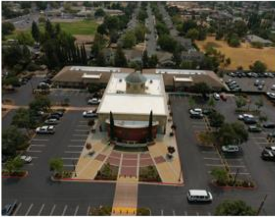
F. Civic Center Roof Replacement Project
