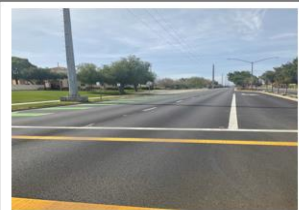
B. Laurel Road Resurfacing Project (O'Hara to Empire)
