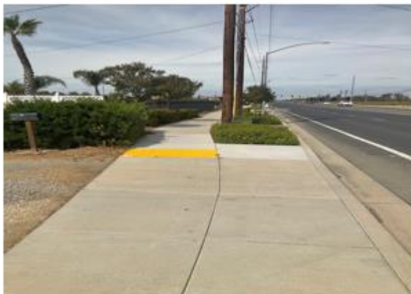
E. Curb, Gutter, & Sidewalk Repair Project
