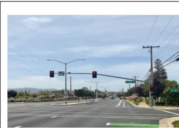
A. Traffic Signal Modernization Project
