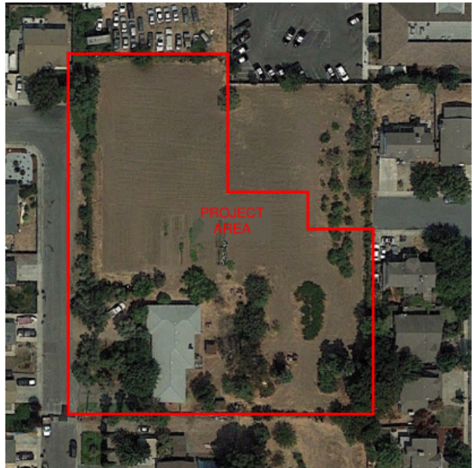
Figure 2. Existing Site Conditions
