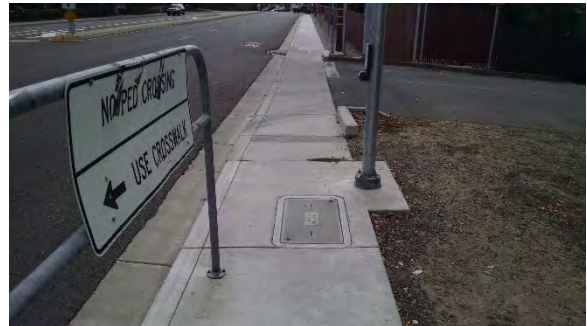
Example of a barrier to pedestrian circulation.
