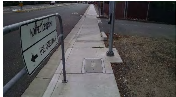
Example of a barrier to pedestrian circulation.
