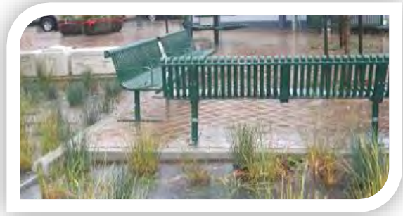
Green stormwater infrastructure is designed to mimic natural processes. This photo shows how landscaped bioretention areas help to detain and slow the flow of stormwater runoff to the storm drain system (Source: Nevue Ngan).
