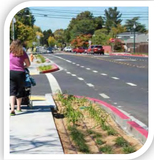
This Sustainable Street in City of San Mateo incorporates a bicycle lane and a “bioretention area” or rain garden that removes pollutants from stormwater runoff (Source: SMCWPPP).
