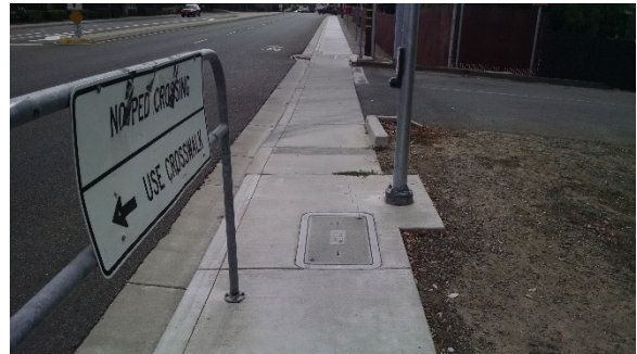
Example of a barrier to pedestrian circulation.
