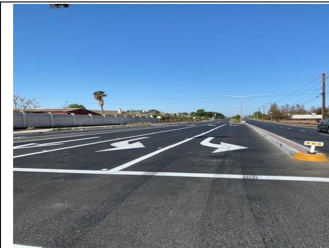
A. Laurel Road Widening (Mellowood to Main)
