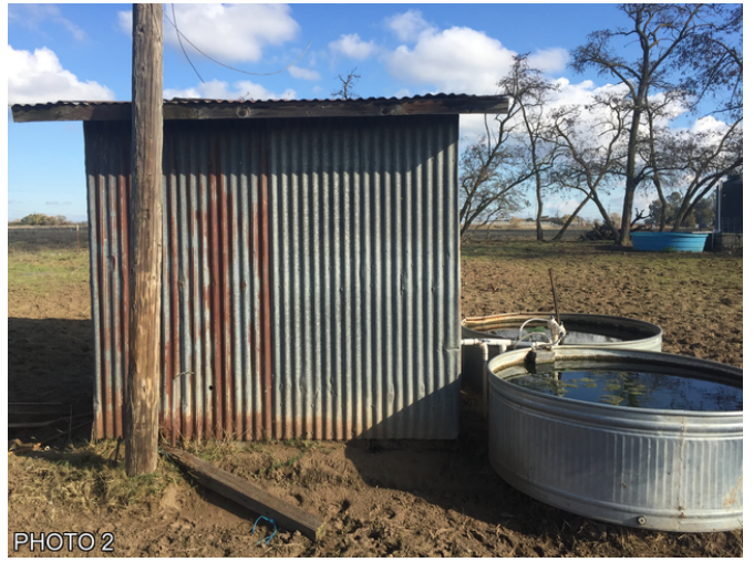
PHOTO 2 VIEW OF WATER TROUGHS AND SHED, LOOKING EAST.
