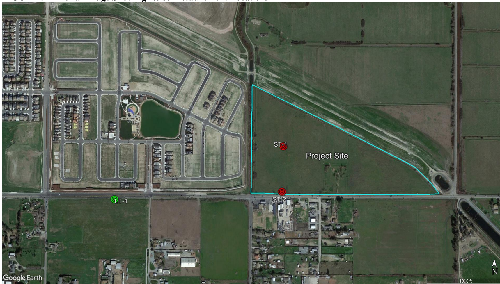
FIGURE 5 Aerial Image Showing Noise Measurement Locations
