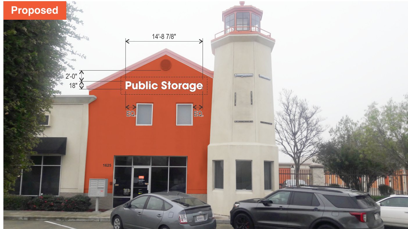
NORTH ELEVATION (OFFICE) -
