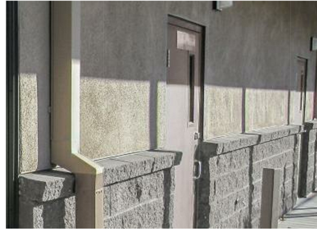
CMU - CONCRETE BLOCK WAINSCOT w/ SILL
