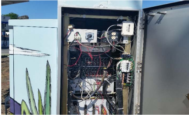
F. FY 2016/17 Traffic Signal Modernization Project
