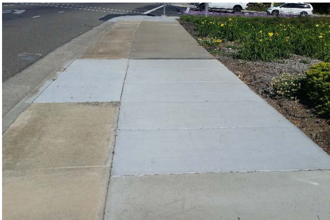
D. FY 2016/17 Curb, Gutter, & Sidewalk Repair and Reconstruction Project
