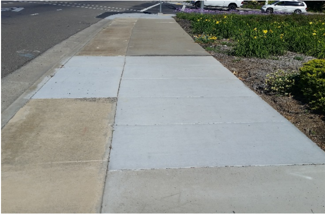
D. FY 2016/17 Curb, Gutter, & Sidewalk Repair and Reconstruction
