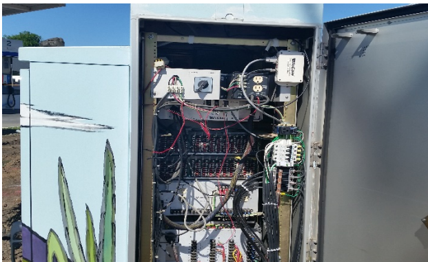
F. FY 2016/17 Traffic Signal Modernization Project
