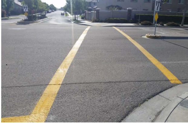
C. FY 2016/17 Street Restriping Project
