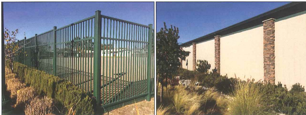
Figure 2. Existing Fencing and Wall
