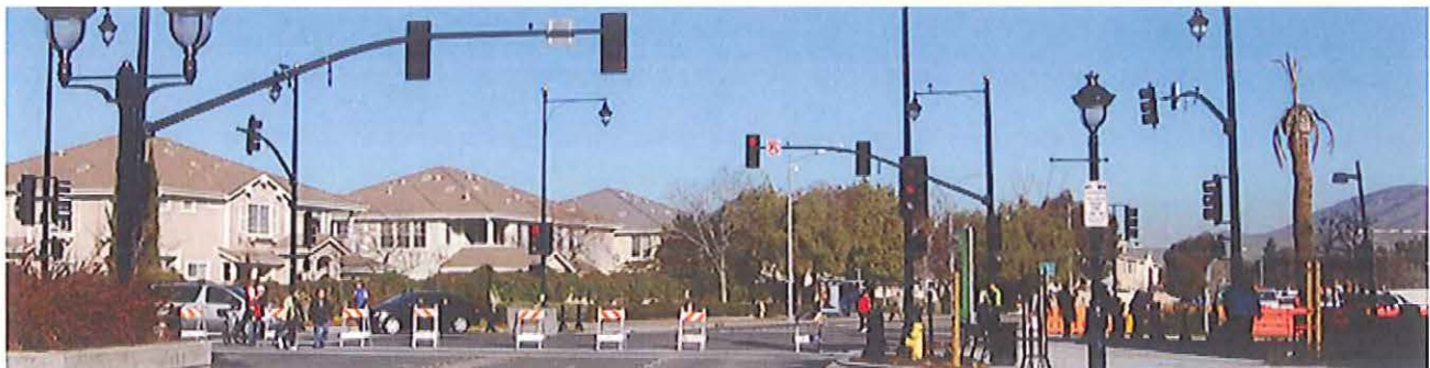
Midtown North Main Street Improvement Project
