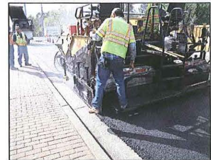
CME'S INSPECTORS WILL TRACK PROGRESS AND PROVIDE SUPERVISION OF CONSTRUCTION ACTIVITIES
