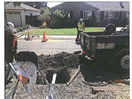
PGE COPPER GAS LINE REPLACEMENT PROJECT PLEASANT HILL, CA
