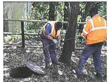
SEWER REPLACEMENT PROJECT PINOLE, CA
