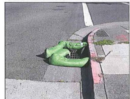
CME HAS STAFF AVAILABLE TO MONITOR SWPPP DURING CONSTRUCTION
