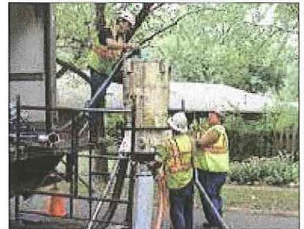
SEWER MAINTENANCE PROJECT PINOLE, CA
