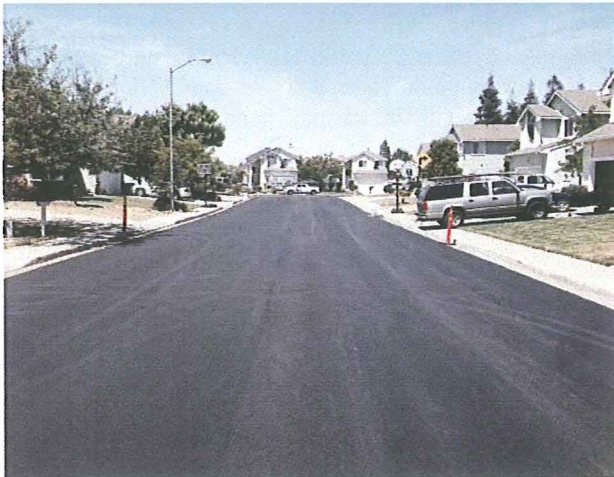
H Pavement Rehabilitation
