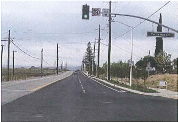
C O'Hara Avenue Widening (Carpenter to Vintage)
