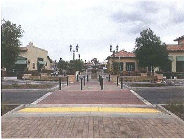
A Main Street Realignment & Downtown Plaza Project
