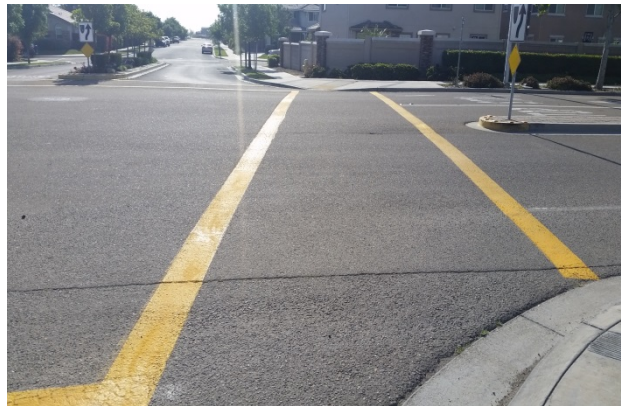
G. City Street Restriping Project
