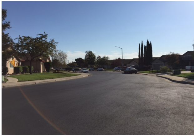
F. Street Repair and Resurfacing Project
