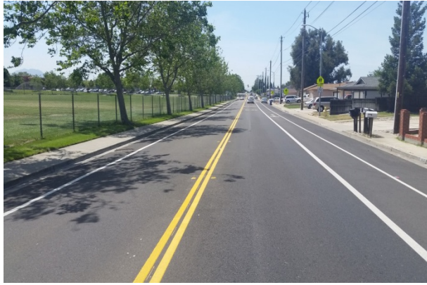
C. Cypress, Big Break & Rose Pavement Rehabilitation Project
