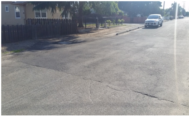
J. Storm Drain Improvement Project
