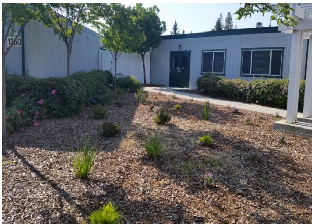
K. ORB Building Rehabilitation Project
