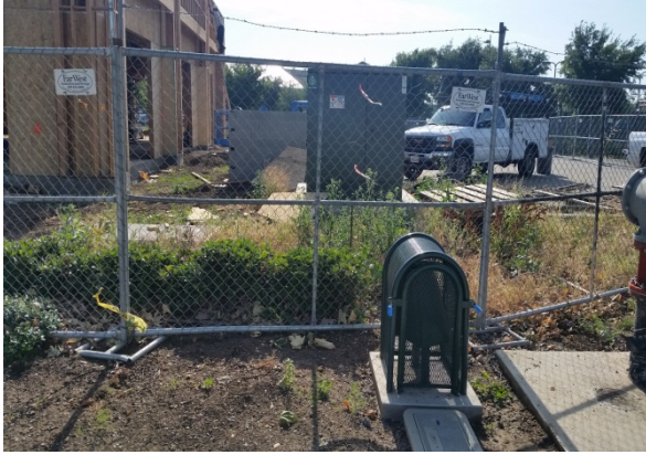
L. Dry Utility Construction at 1530 Neroly Road
