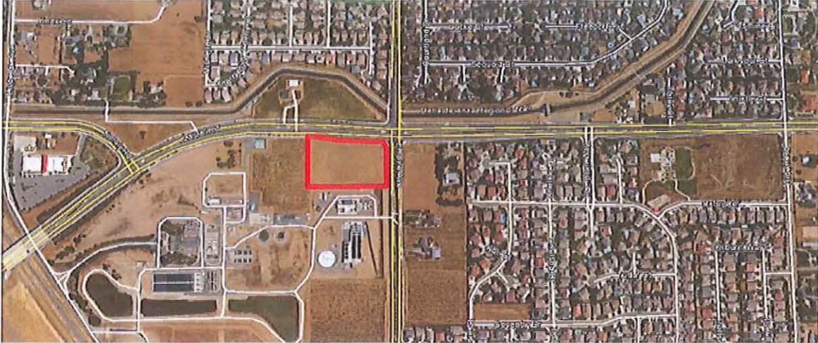
Figure 2. Aerial of Project Site and Adjacent Properties
