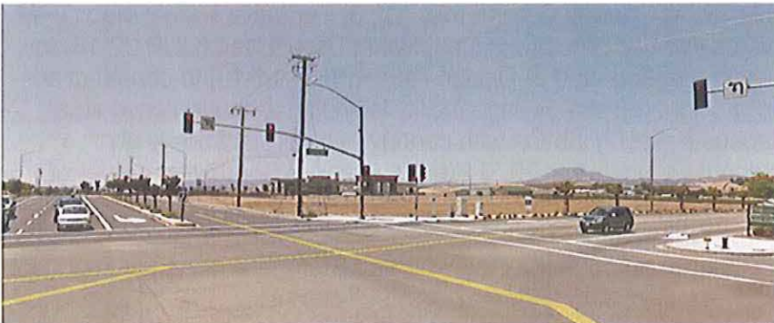
Figure 1. Street View of Project Site
