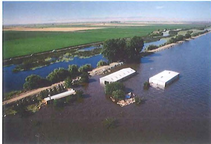
DWR Photos: June 2004 Jones Tract Breach and Flood
