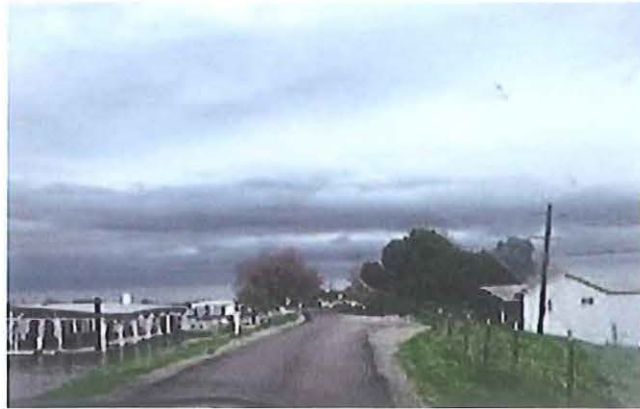
GJ photos: Pictures of levee crowns
