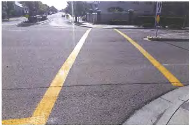
G. City Street Restriping Project
