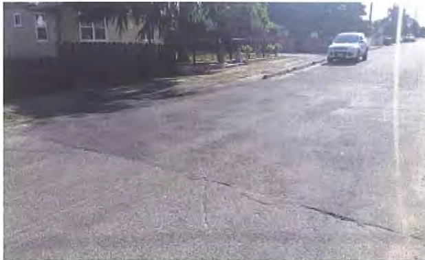
J. Storm Drain Improvement Project
