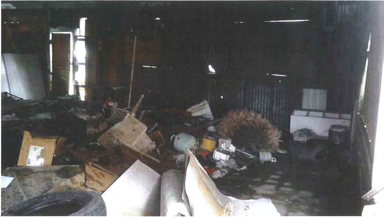
150 E Acme Trash and Building Materials from Exterior of Property Moved Inside
