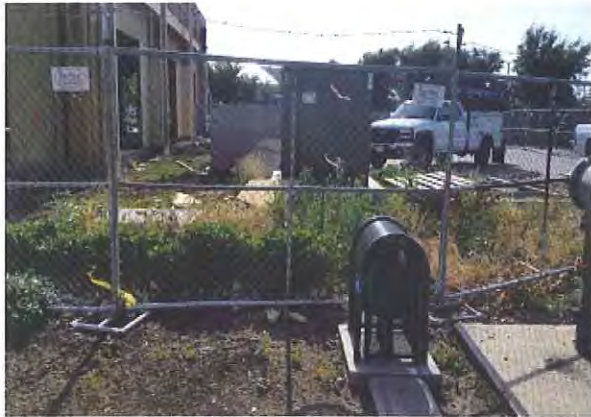
L. Dry Utility Construction at 1530 Neroly Road
