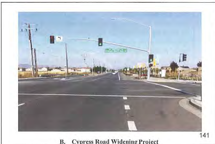
B. Cypress Road Widening Project
