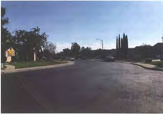
F. Street Repair and Resurfacing Project
