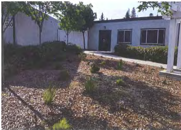
K. ORB Building Rehabilitation Project
