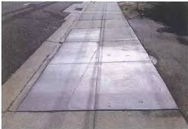
H. Curb, Gutter, & Sidewalk Repair and Reconstruction Project
