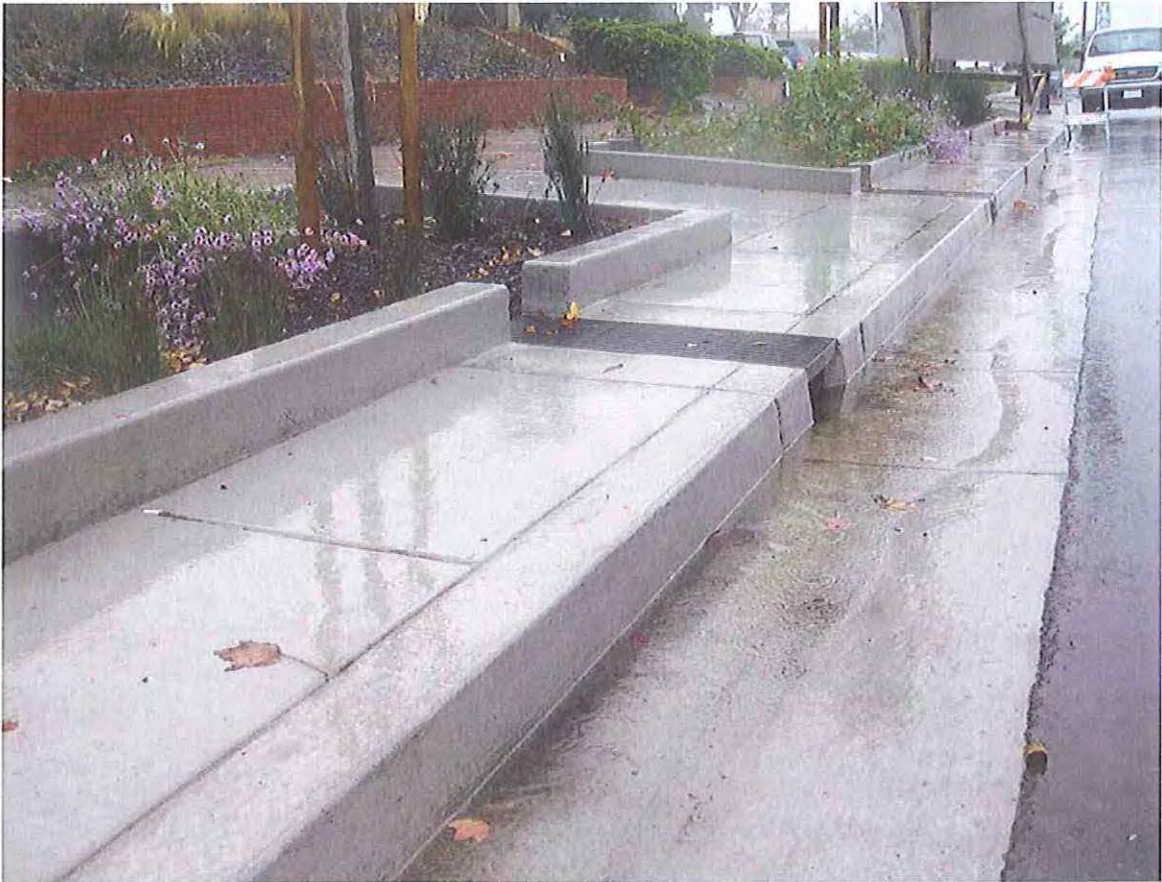
Green Infrastructure: Bioretention facilities treating street runoff.
