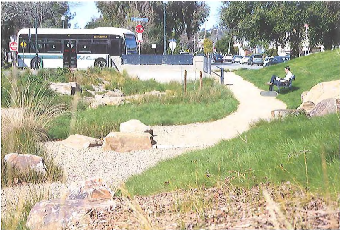
Green Infrastructure: Bioretention facility with active and passive landscape uses (El Cerrito)
