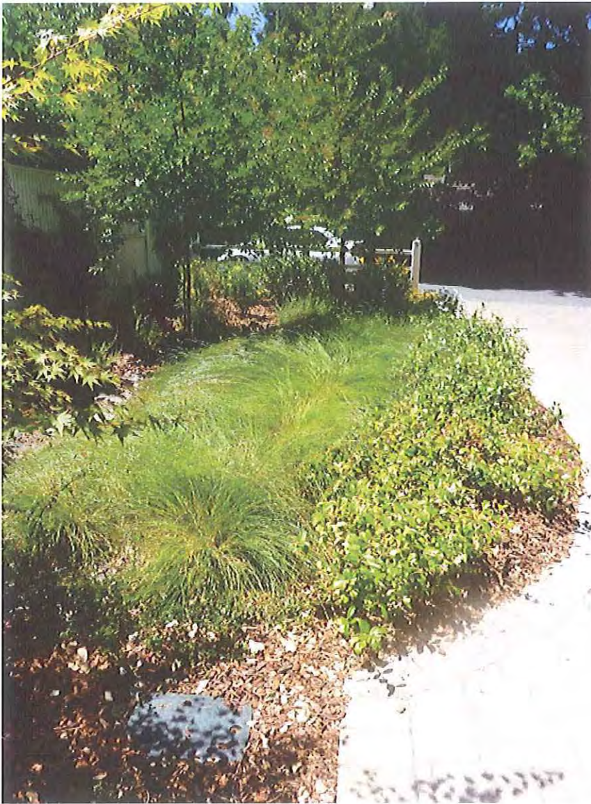
Green Infrastructure: Bioretention treating runoff from residences and a private street (Contra Costa County)
