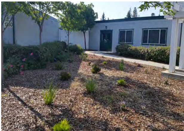
K. ORB Building Rehabilitation Project
