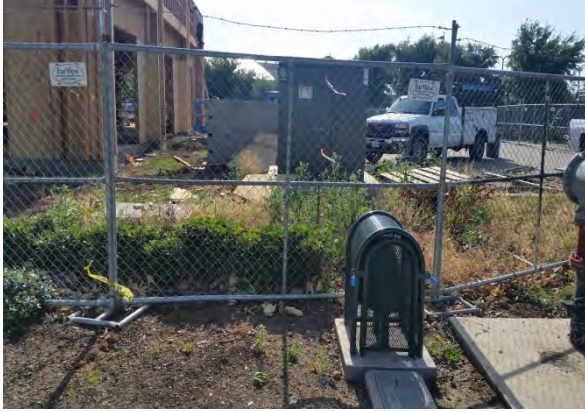
L. Dry Utility Construction at 1530 Neroly Road
