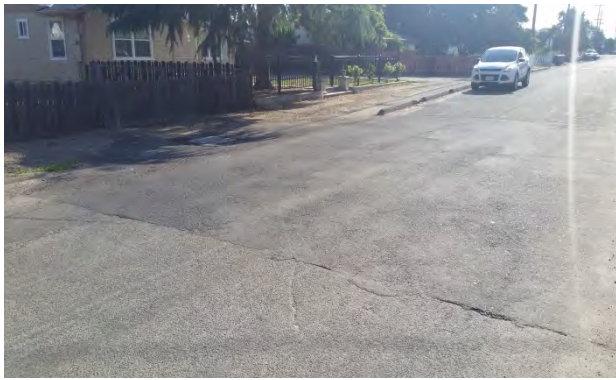
J. Storm Drain Improvement Project
