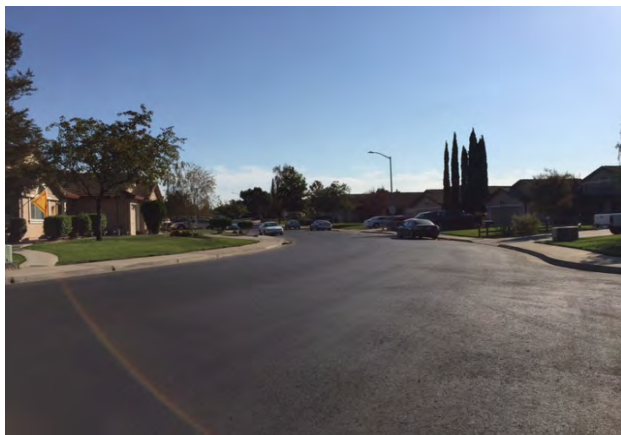
F. Street Repair and Resurfacing Project
