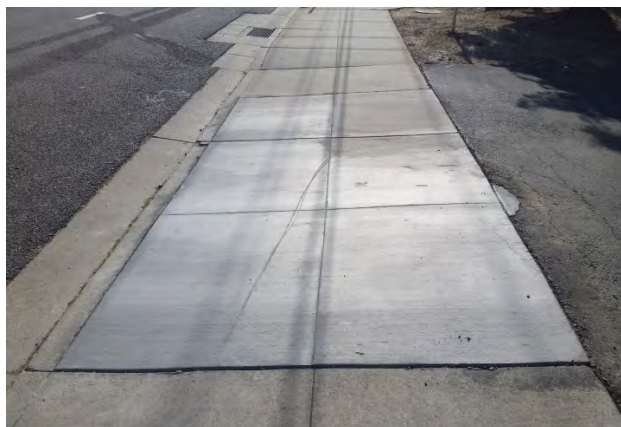
H. Curb, Gutter, & Sidewalk Repair and Reconstruction Project
