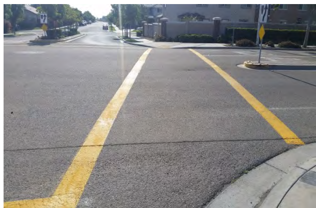
G. City Street Restriping Project
