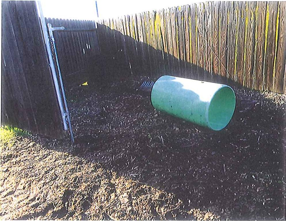
This is a short piece of the new 24" pipe that was placed inside the existing storm drain pipe.
