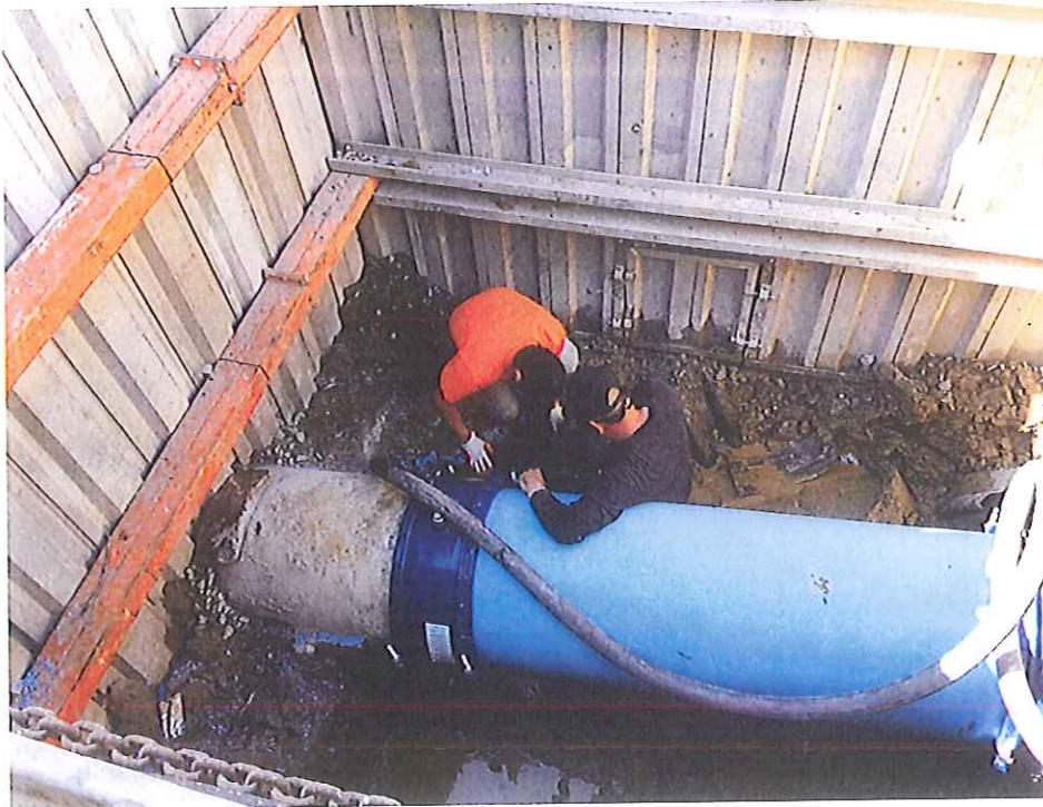
The crew is pumping concrete into the space inside the old storm drain pipe to seal it with the new pipe inside.
