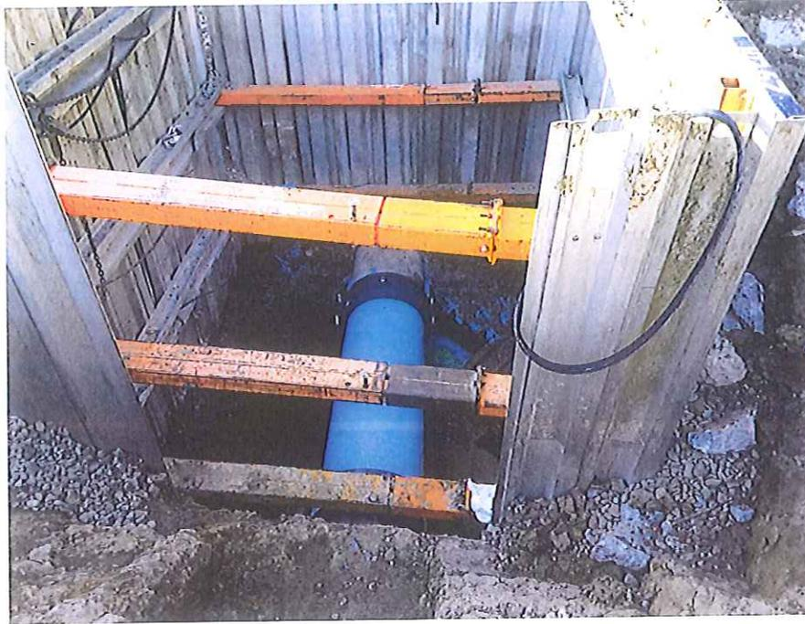
The new section of water pipe is in place as is the new storm drain pipe inside of the old pipe.
