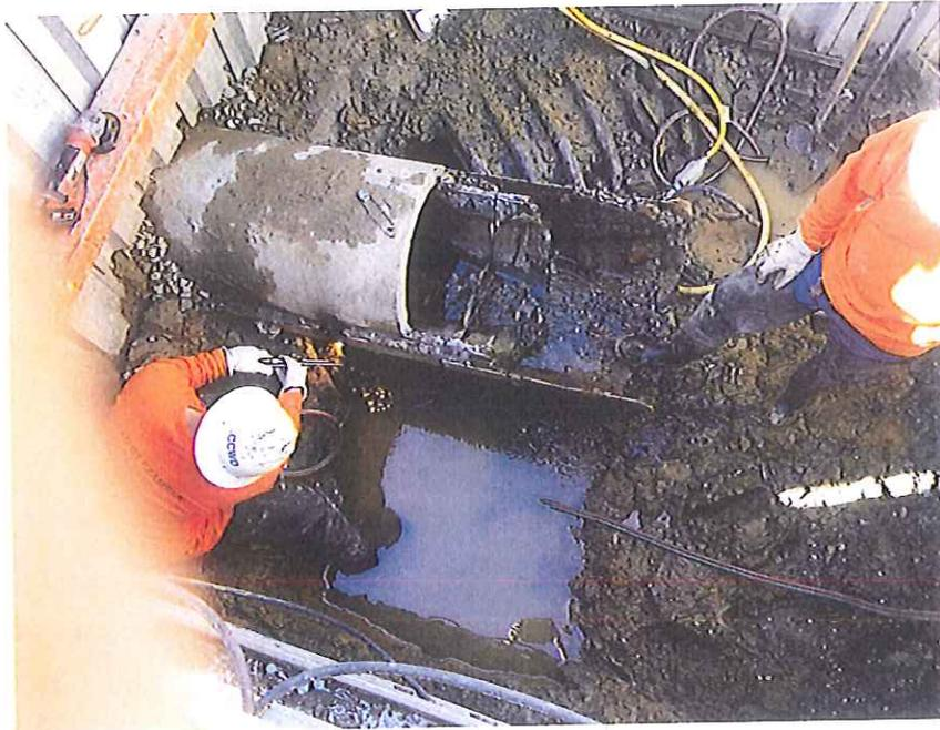
The CCWD water pipe has been partially removed and the hole in the storm drain pipe is visible on both side of the water pipe.
