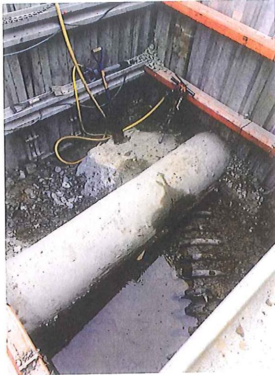
The CCWD water pipe is on top of the storm drain pipe and the hole in the storm drain pipe is partially visible.
