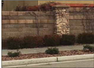
8' HEIGHT PROJECT SOUND WALL TO MATCH EXISTING SOUND WALL ON ADJACENT PROPERTY
