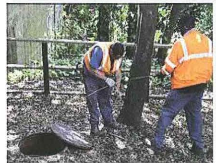
SEWER REPLACEMENT PROJECT PINOLE, CA
