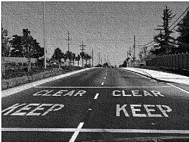
H City Street Restriping Project
