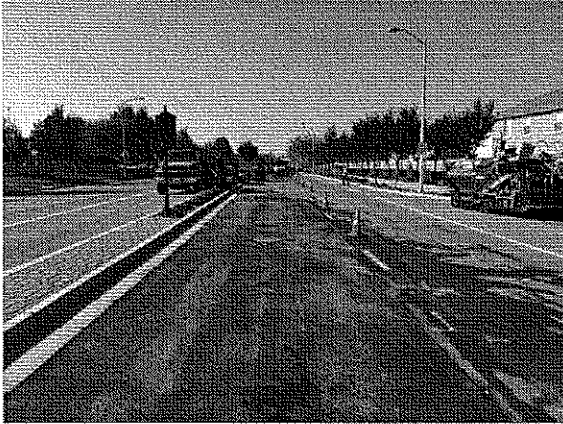
C Street Resurfacing and Repair Project
