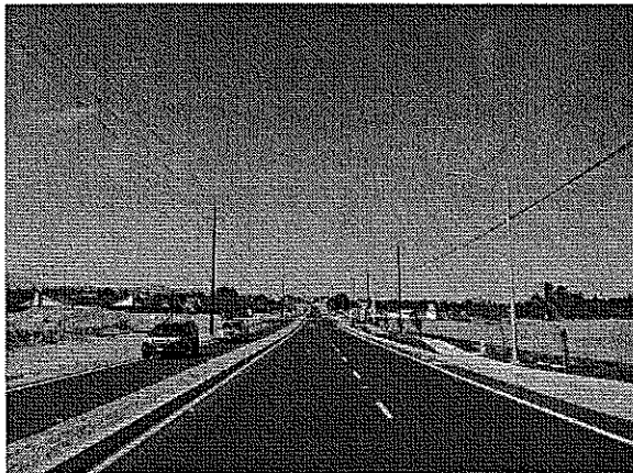
F Laurel Road Widening Project
