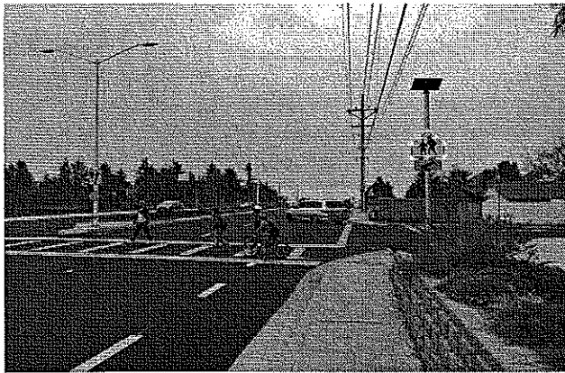
E Traffic Safety Improvement Project
