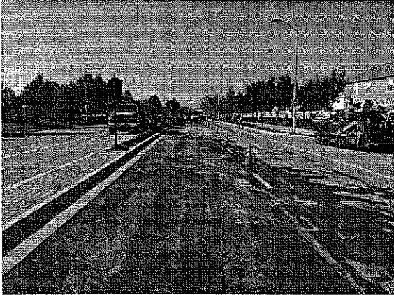
C Street Resurfacing and Repair Project
