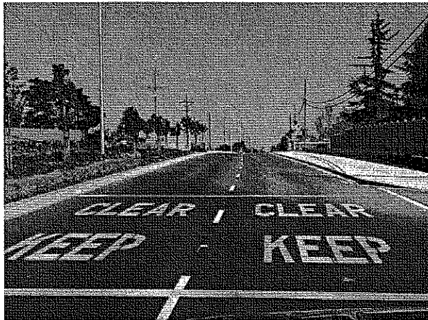
H City Street Restriping Project
