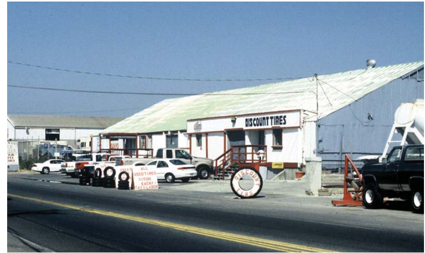
The appearance of Downtown buildings and street frontages need to be significantly improved. Auto services will not remain part of Downtown Oakley’s land use mix.
