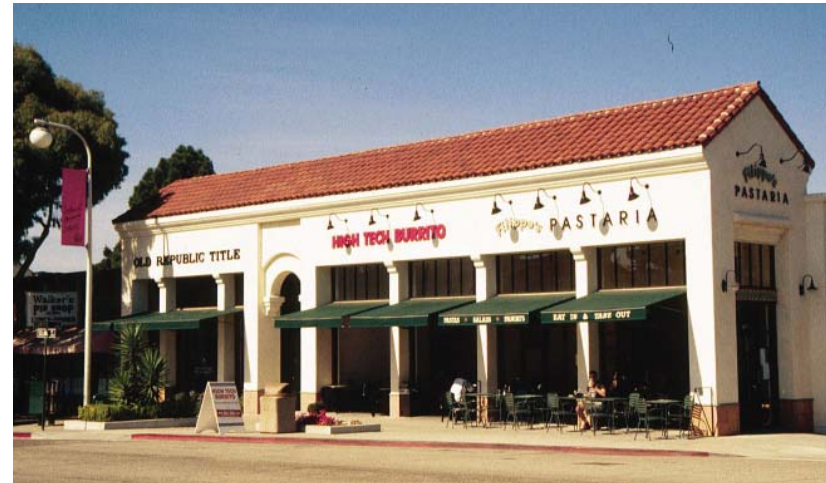
Highlighting building bays with pilasters adds interest to a simple building form.
