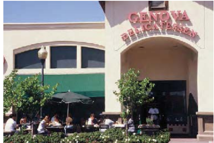
Signs should be located on prominent building forms. Pole-mounted signs are discouraged.
