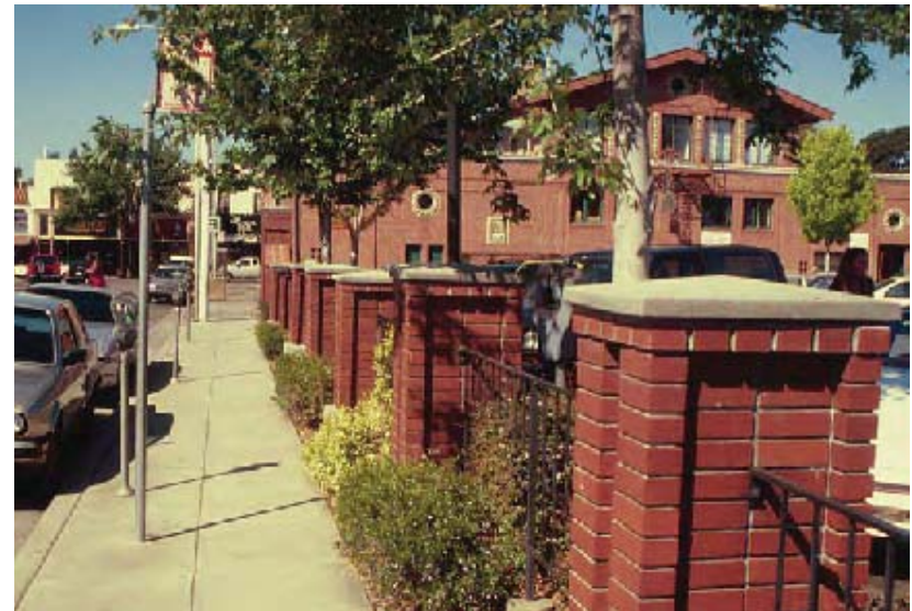
This combination of brick piers and open fencing complements the principal building and screens the adjacent parking lot.
