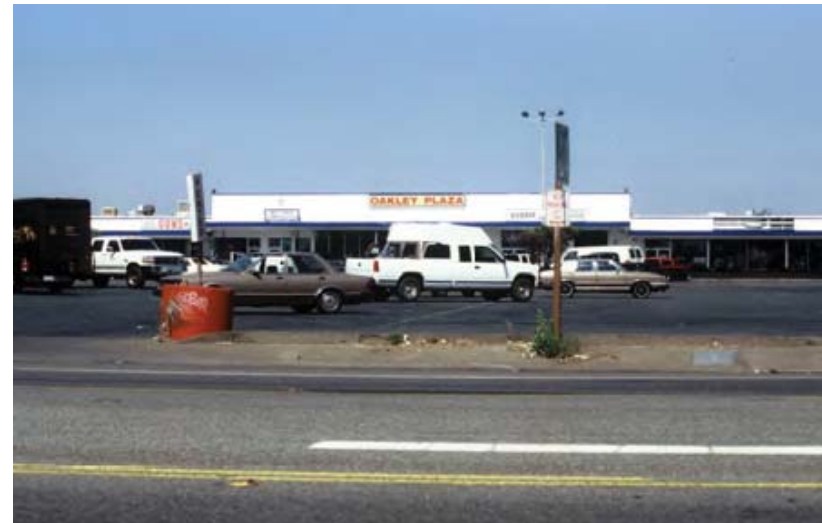
One story buildings and surface parking in Oakley
