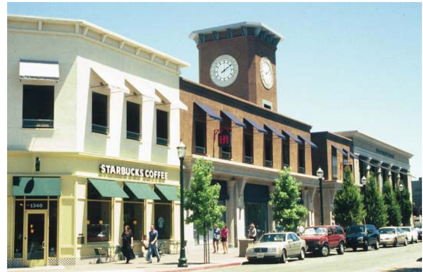
Structured parking is provided on the second and third floors of this Walnut Creek commercial development.
