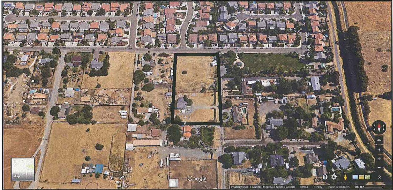
Figure 1. Aerial Photo of Project Site
