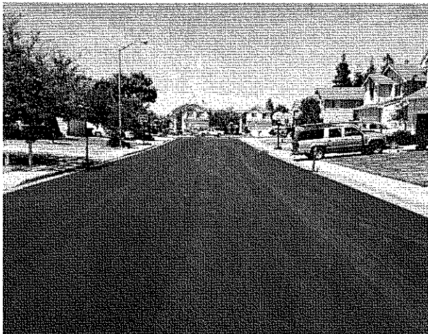
H Pavement Rehabilitation
