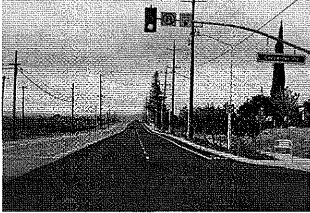
C O'Hara Avenue Widening (Carpenter to Vintage)
