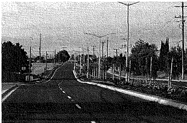
B O'Hara Avenue Widening (Covered Wagon to Laurel)
