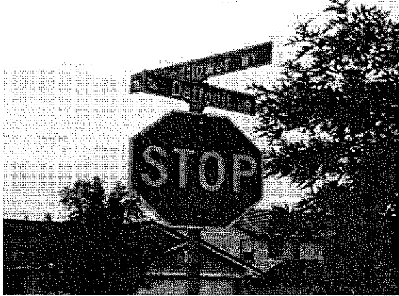
F Citywide Street Name Sign Replacement Project
