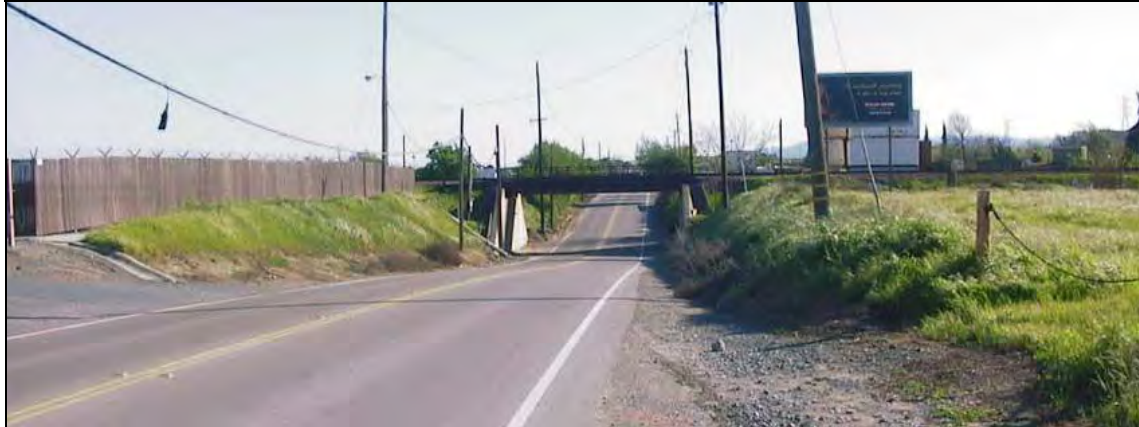
Figure 2-14 View South Along Bridgehead Road at Railroad Crossing
