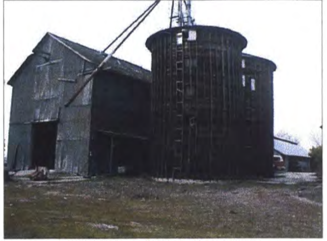
BARN/SILOS - BURROUGHS DAIRY
